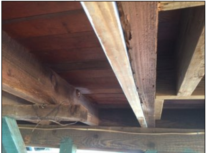
Termite damage and evidence of repairs.
