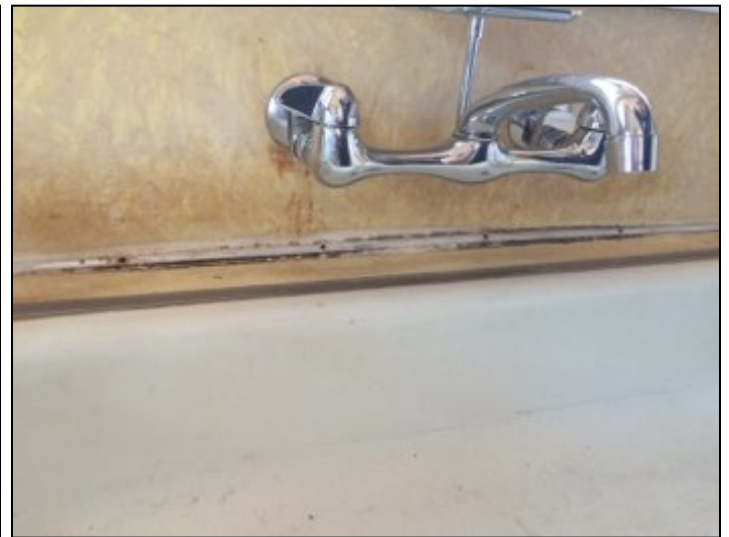
Deteriorated caulking at kitchen countertop.
