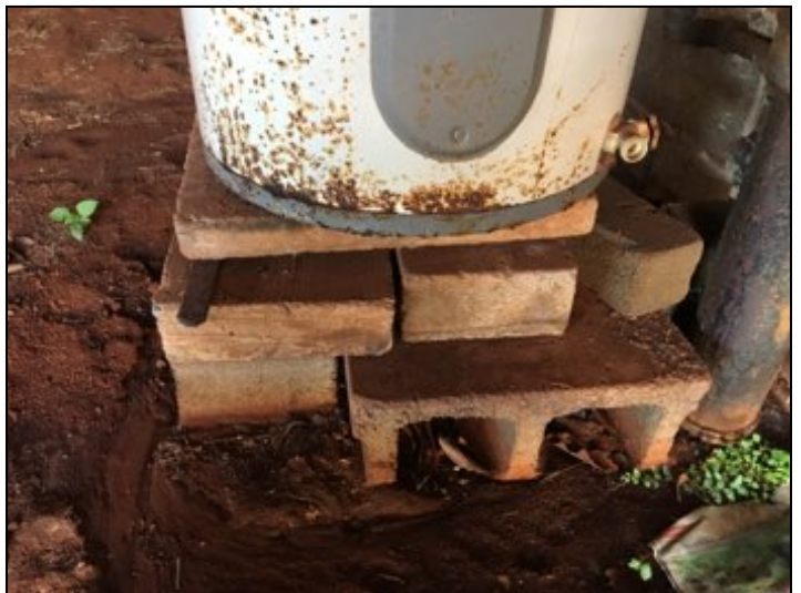
Significant rust at water heater base. Improper water heater platform.
