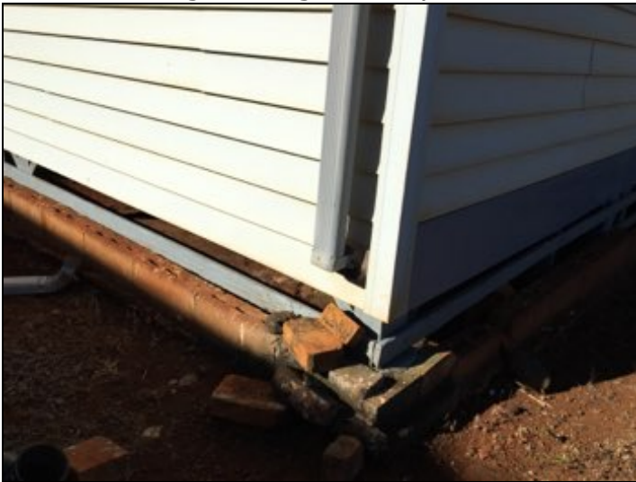
Rain gutter downspout missing components.
