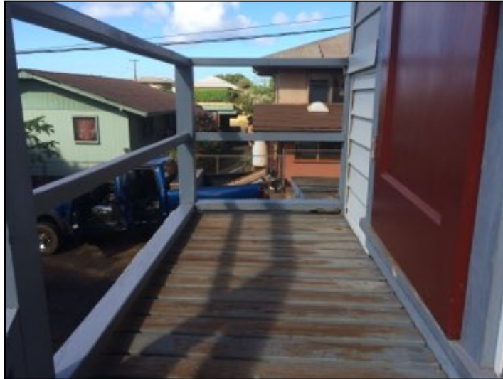
Safety rail does not meet current safety standards.
