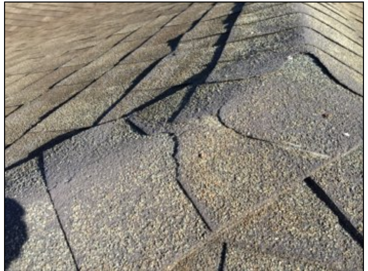
Damaged roof shingles.
