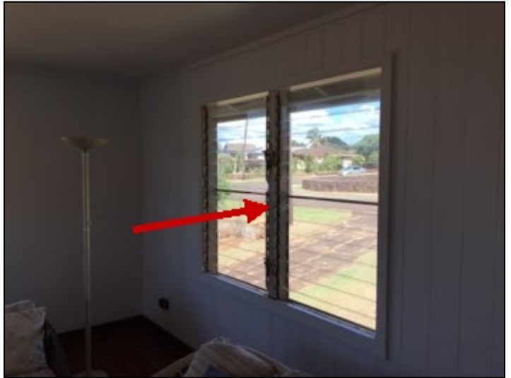
Termite damage at window frame.
