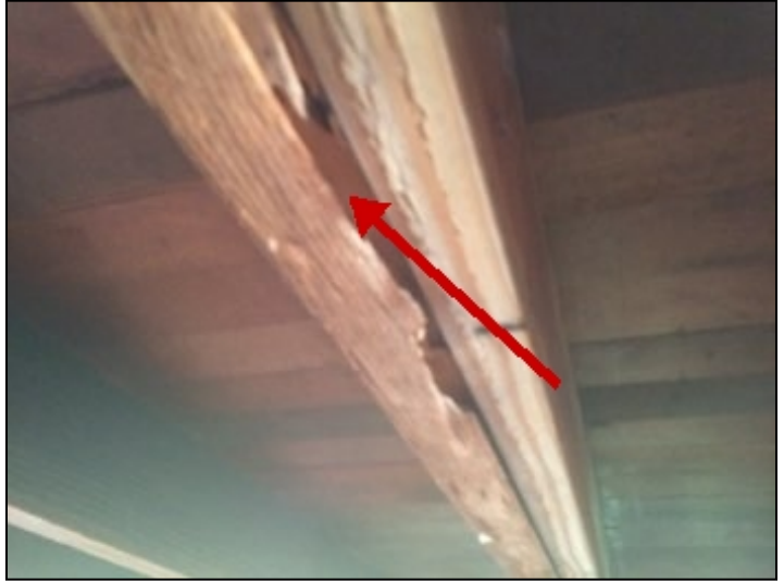
Termite damage and evidence of repairs.
