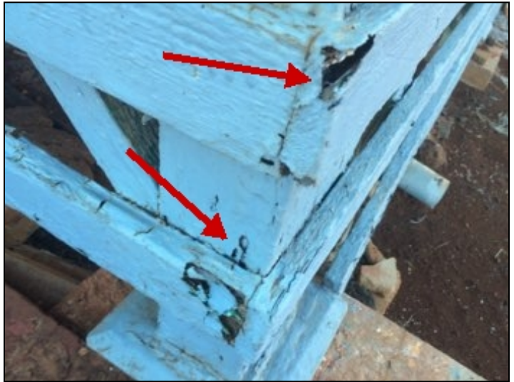
Significant termite damage to skirting and foundation post at the front of home.
