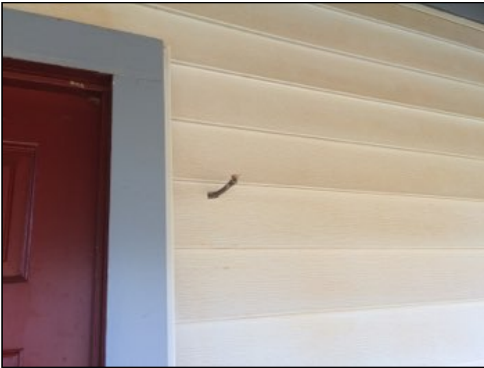
Missing light fixture, bare wires at main entry door.
