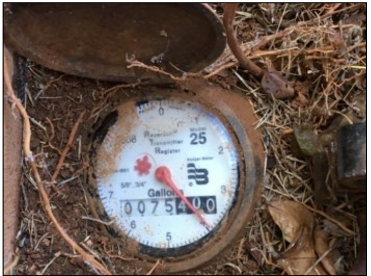
Water meter registers water use with no fixtures in use.
