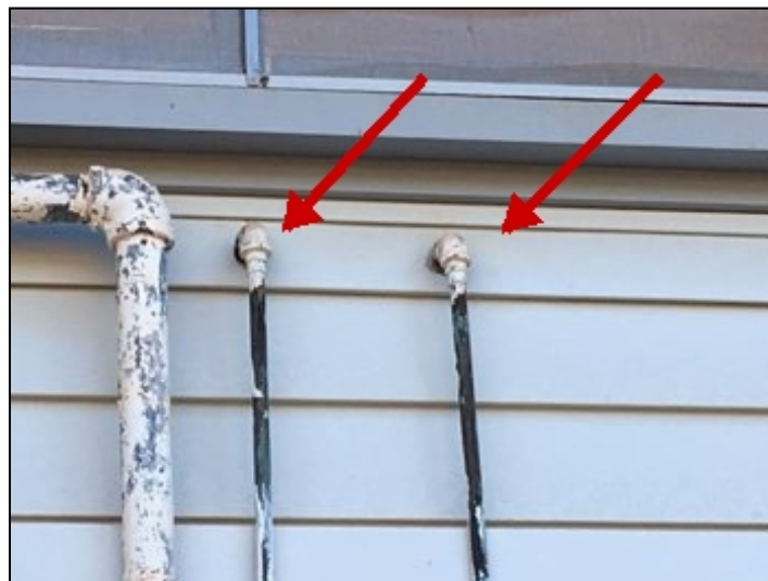
Galvanized pipe connected directly to copper pipe.
