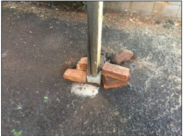
Significant damage/ improper construction.
