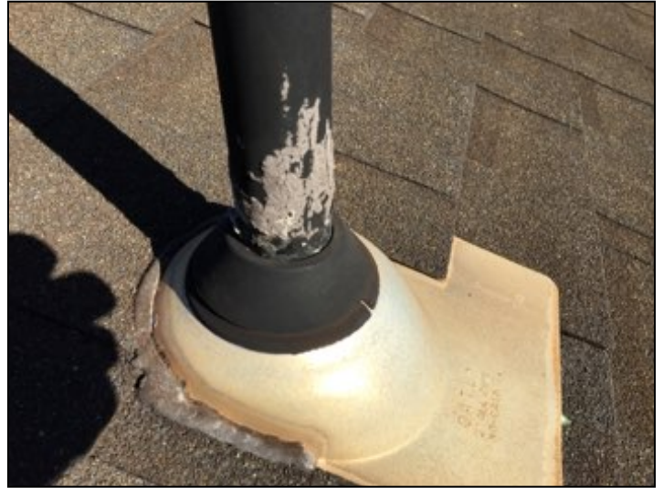
Deteriorated rubber gaskets at plumbing vents.
