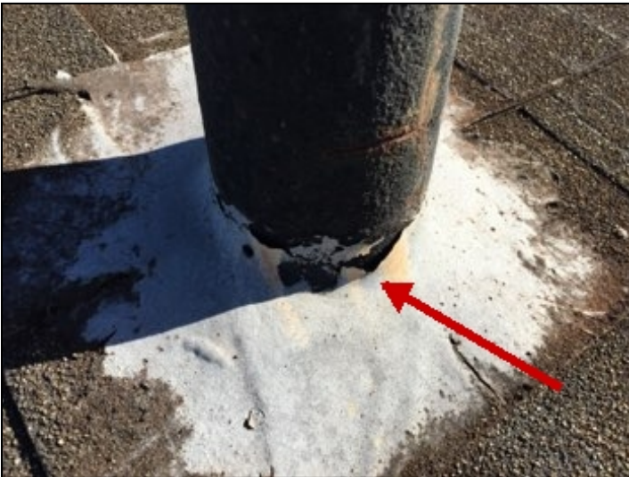
Deteriorated sealant.
