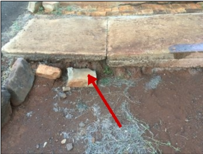
Soil subsidence at front walkway.
