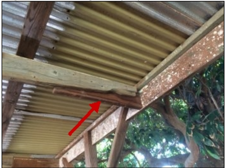
Improper repairs.
