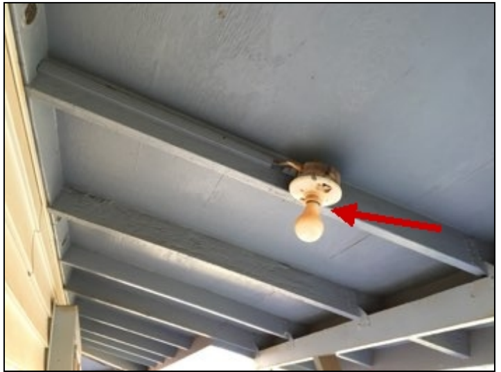
Light bulb arcing at socket.
