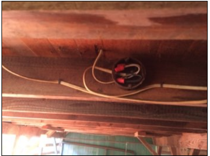
Open electrical junction boxes at foundation.
