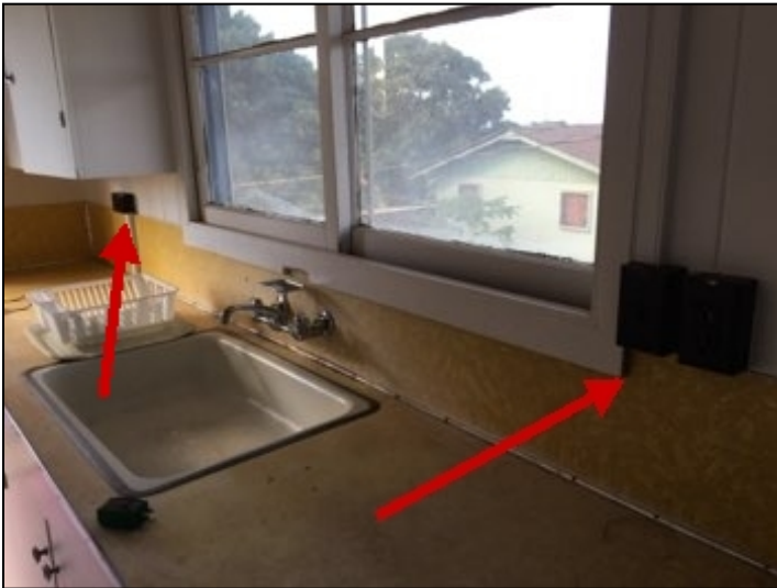
No GFI protected receptacles at kitchen sink.
