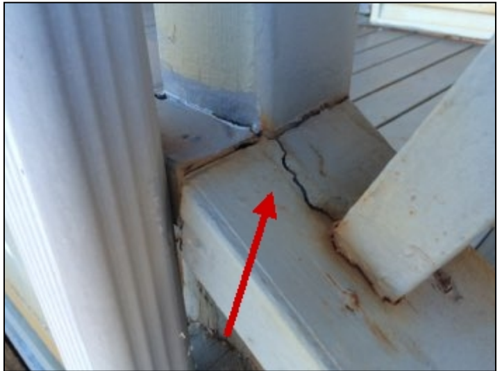
Deterioration at entry stair handrail.
