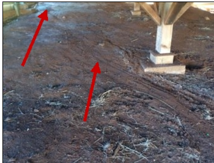
Evidence of moisture from poor drainage.
