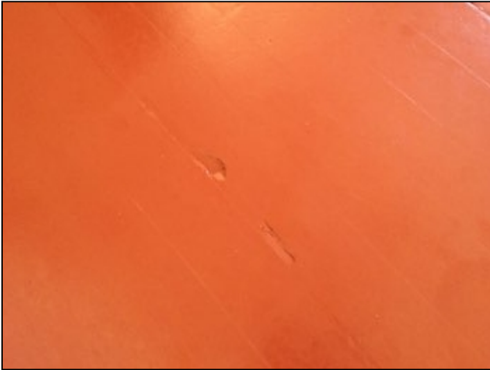
Termite damage at kitchen floor.
