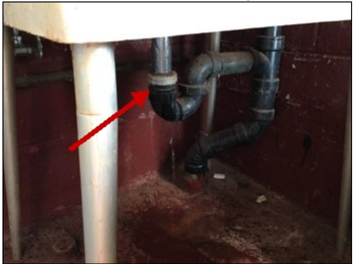
Lower level utility sink leaks at trap.
