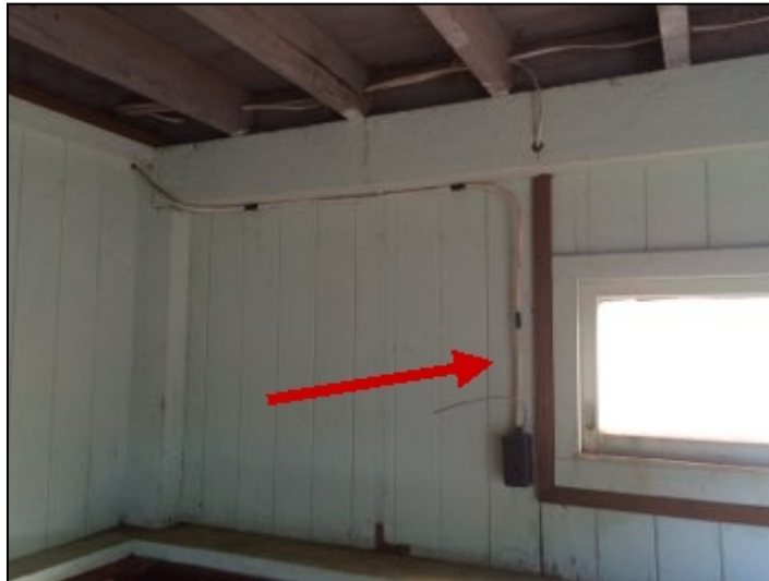
Exposed romex wires.
