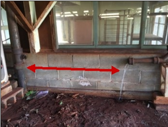
Missing section of plumbing drain pipe.
