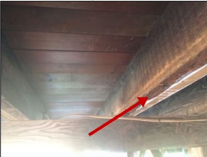
Termite damage and evidence of repairs.
