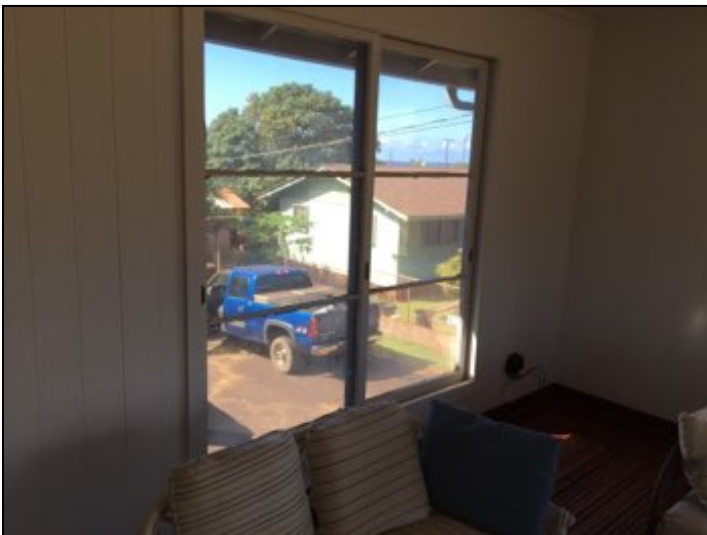
Living room window height does not meet current safety standards.
