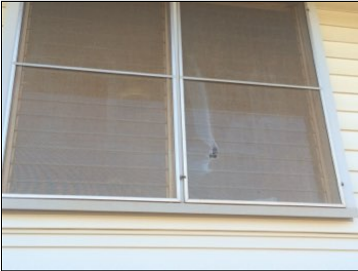
Damaged window screen west side of home.
