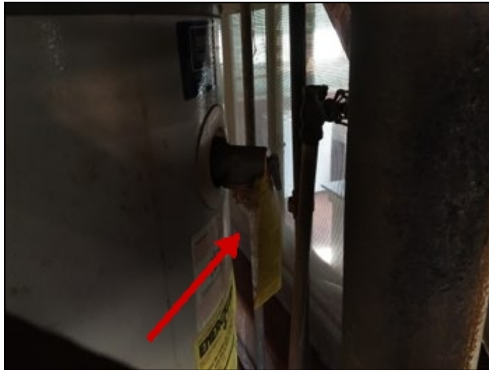
Missing TPR valve extension.
