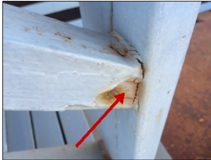
Deterioration at entry stair handrail.
