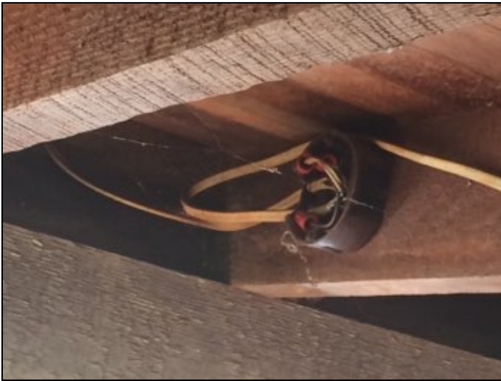
Open electrical junction boxes at foundation.
