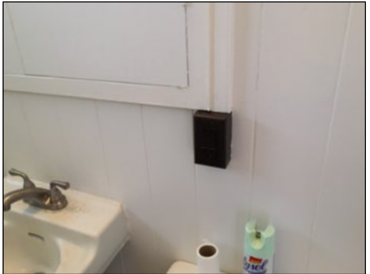
GFI outlet in bathroom did not respond to test.
