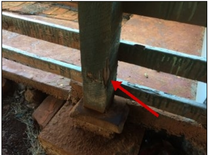
Termite damage.
