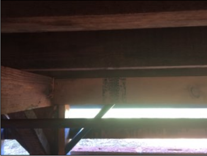
Evidence of repairs at foundation.
