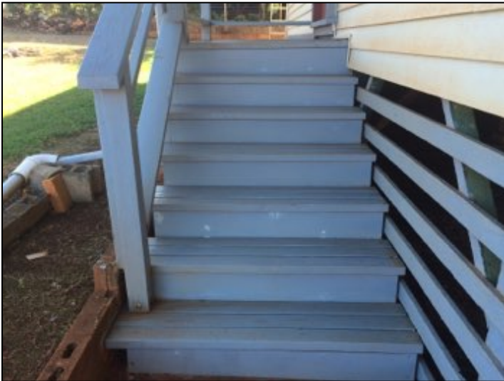
Front entry stairs.
