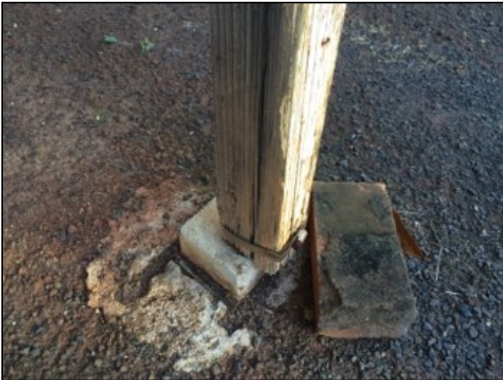
Significant damage/ improper construction.
